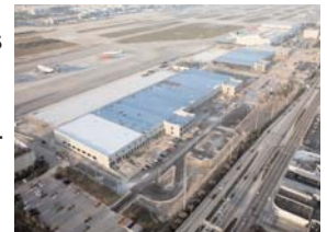
Centurion Air Cargo Facility
